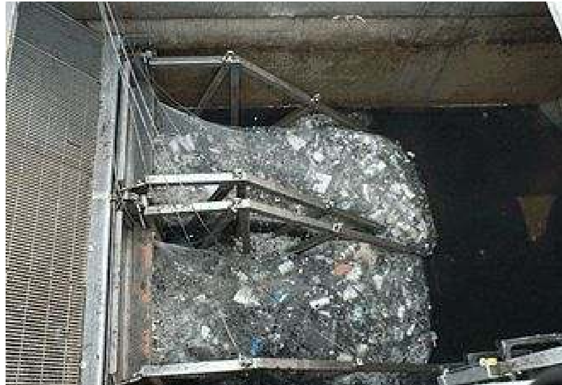
Fresh Creek Technologies Netting Trash Trap
