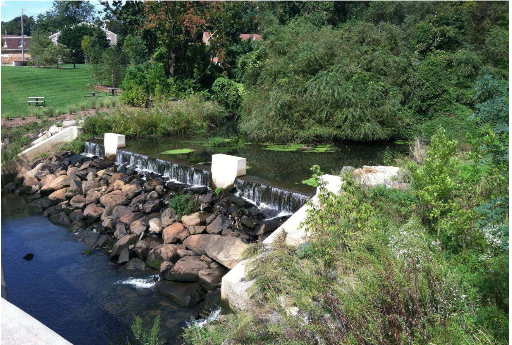
Raise concrete weir and installation of stop logs proposed at outfall to increase water level within Mill Pond.
